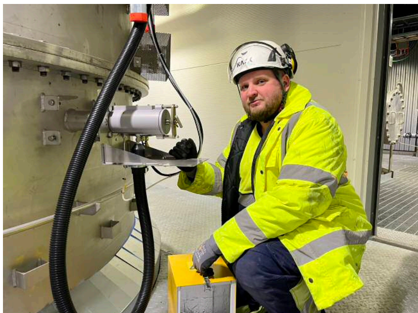
Service technician Anders Hinders from OPSIS takes a closer look at the probe mounted on the flue gas duct.
