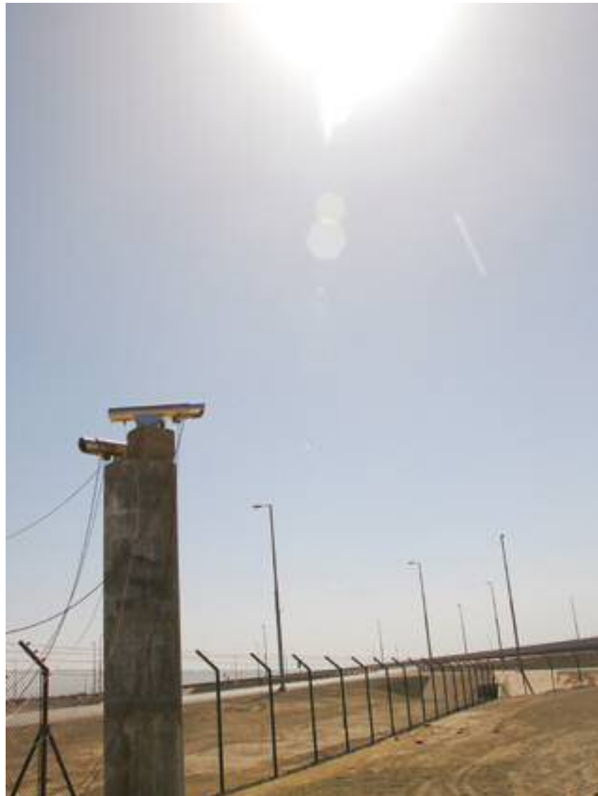
Fence-line monitoring at Sohar Port, Oman.
